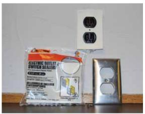
Sealing air leaks in manufactured homes can help lower utility costs. Installing foam outlet gaskets behind electrical outlets and light switches is just one way to help save energy.
